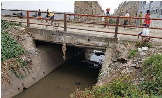
Figure 2-33: Hola road bridge
