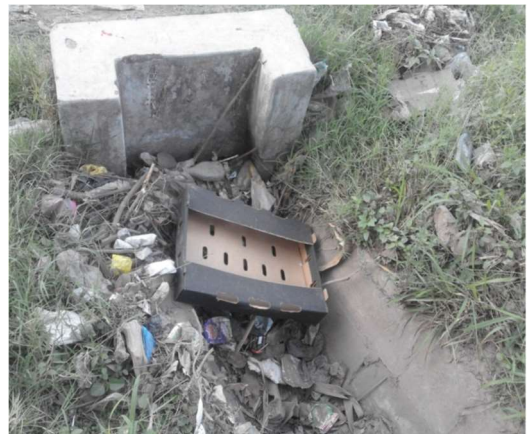
Figure 2-36: Blocked culvert
