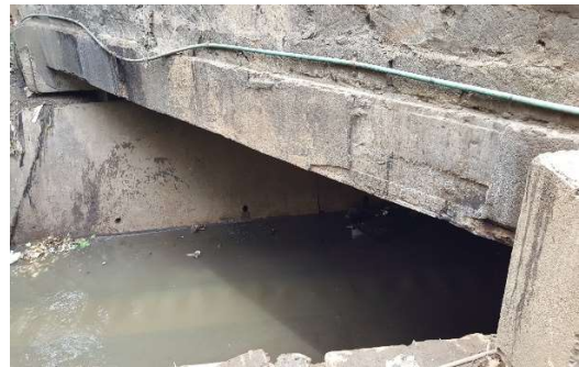
Figure 2-34: Shimo la tewa road bridge
