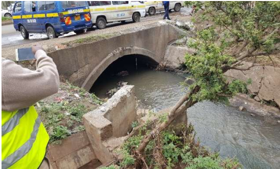
Figure 2-31: Bunyala road culvert
