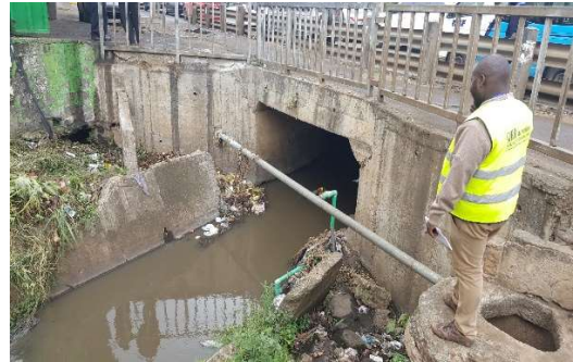
Figure 2-32: Lusaka road culvert
